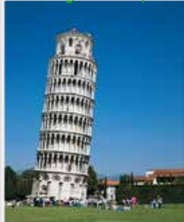
Leaning Tower of Pisa
